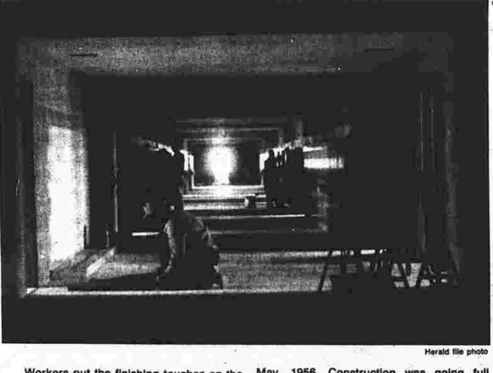
Workers put the finishing touches on the underneath section of the new high school in May, 1956. Construction was going full speed ahead that spring.
